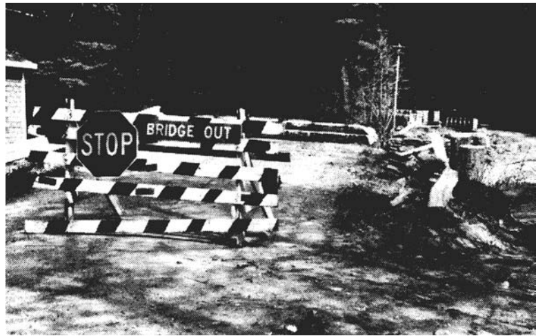
Graham Road Bridge Repair
