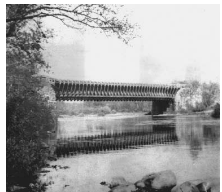
Roebling Neversink Aqueduct
