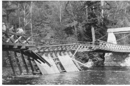
An overloaded truck caused this collapse of the Godeffroy bridge in 1927.
