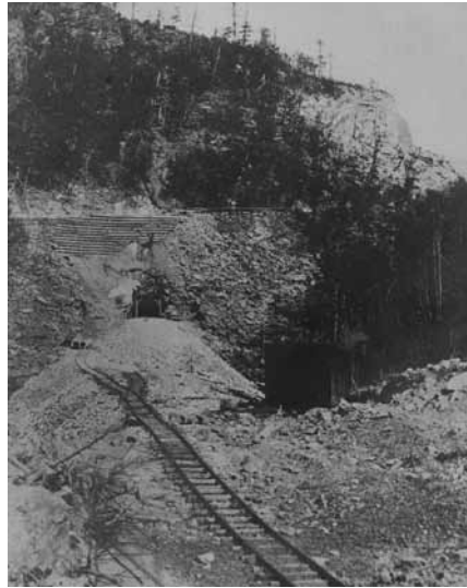
Otisville Tunnel—Western Portal a private enterprise, the Erie." *
