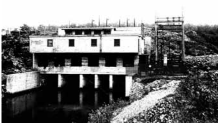
Hydro-Electric Power Plant Hoag Road Cuddebackville, NY John Lewis Oral History
