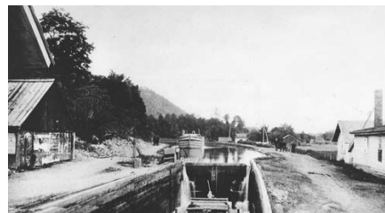
D & H Canal Lock 56 Photo Deerpark Historian’s Office
