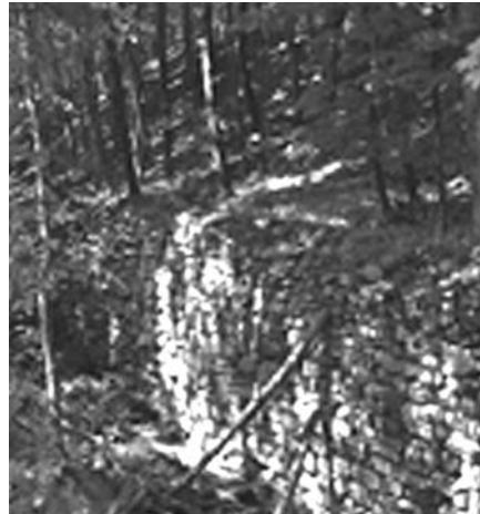
Original D & H Canal stonework along the Trail. All work was done with hand tools and no mortar to hold the stones.
