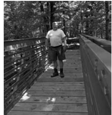
Cliff Robinson and the new 60’ bridge spanning a breach in the D & H Towpath Trail
