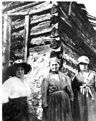
This picture of a log house, on Prosper Davis Road, Rio, is the only one available showing the construction of early homes in this area. The woman in the center is a Delaware Indian, Iantha Jacoby Davis Marshall. (year of photo unknown). Prosper Davis Road was named for Prosper Davis (1804-1888) who was married to Viola Jacoby (1851-1942). The town of Forestburgh requested that the road be closed, however Deerpark turned down the request because the parcels of land located on the road would have been landlocked. Photo recorded by Richard Carey, former Deerpark Historian.
